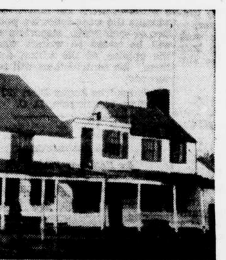
Rear view of the Anton Ruppert house, Bladensburg road.
