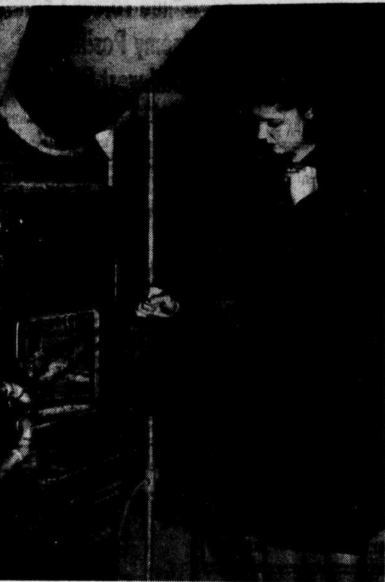
Lady stokers should never forget the "bright spot." Gently pull a few live coals to the front of the firebox and leave them uncovered when you add fresh coal. The "bright spot" helps ignite the new coal and burn up gases.
