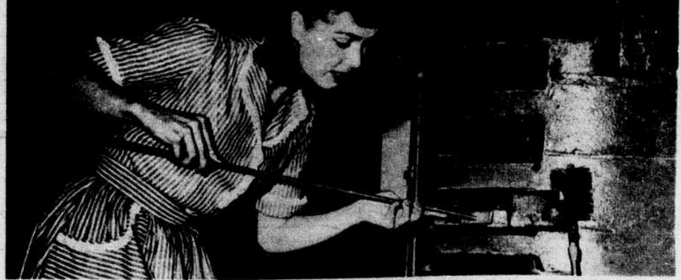
1. She begins by opening clean-out door and removing dust ash
