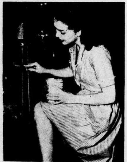
4. With furnace cement, she stops leaks that waste coal
