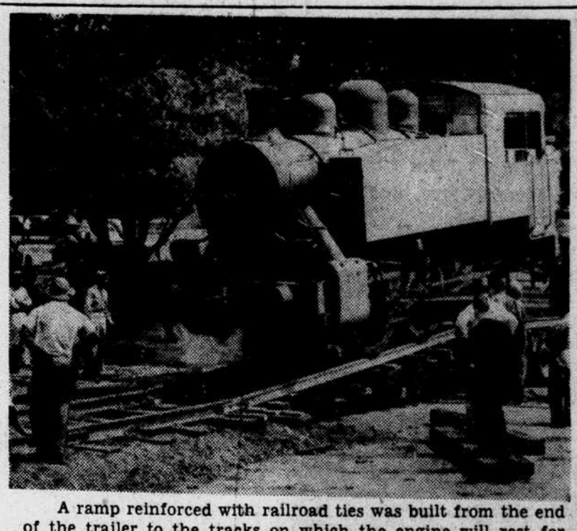
A ramp reinforced with railroad ties was built from the end of the trailer to the tracks on which the engine will rest for public inspection. Here the engine descends the ramp.
