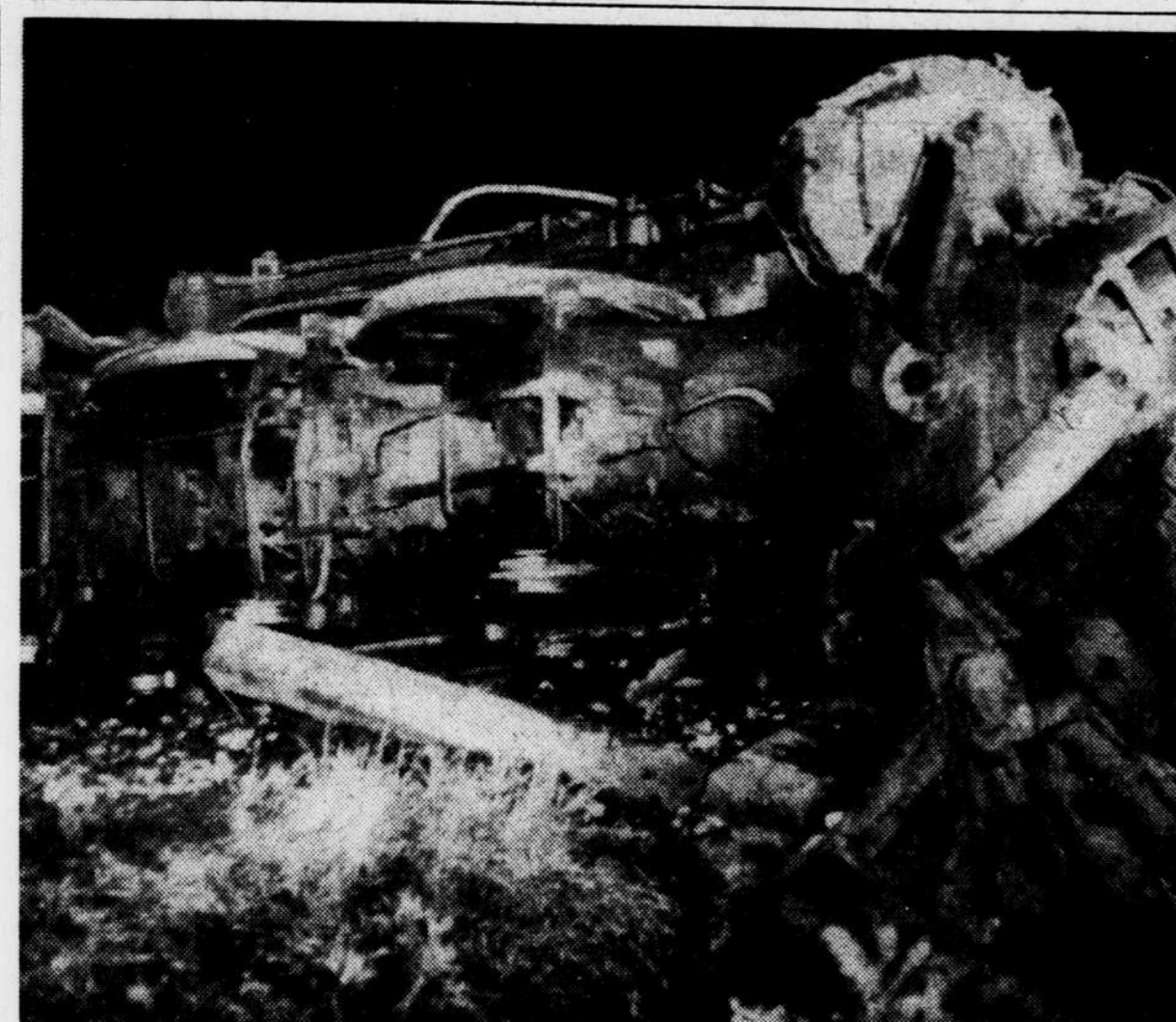
WAYLAND, N. Y.—SCENE OF FATAL TRAIN CRASH—This twisted mass of wreckage is the engine of the Delaware, Lackawanna & Western's Lackawanna limited which collided with a freight engine near here today.
