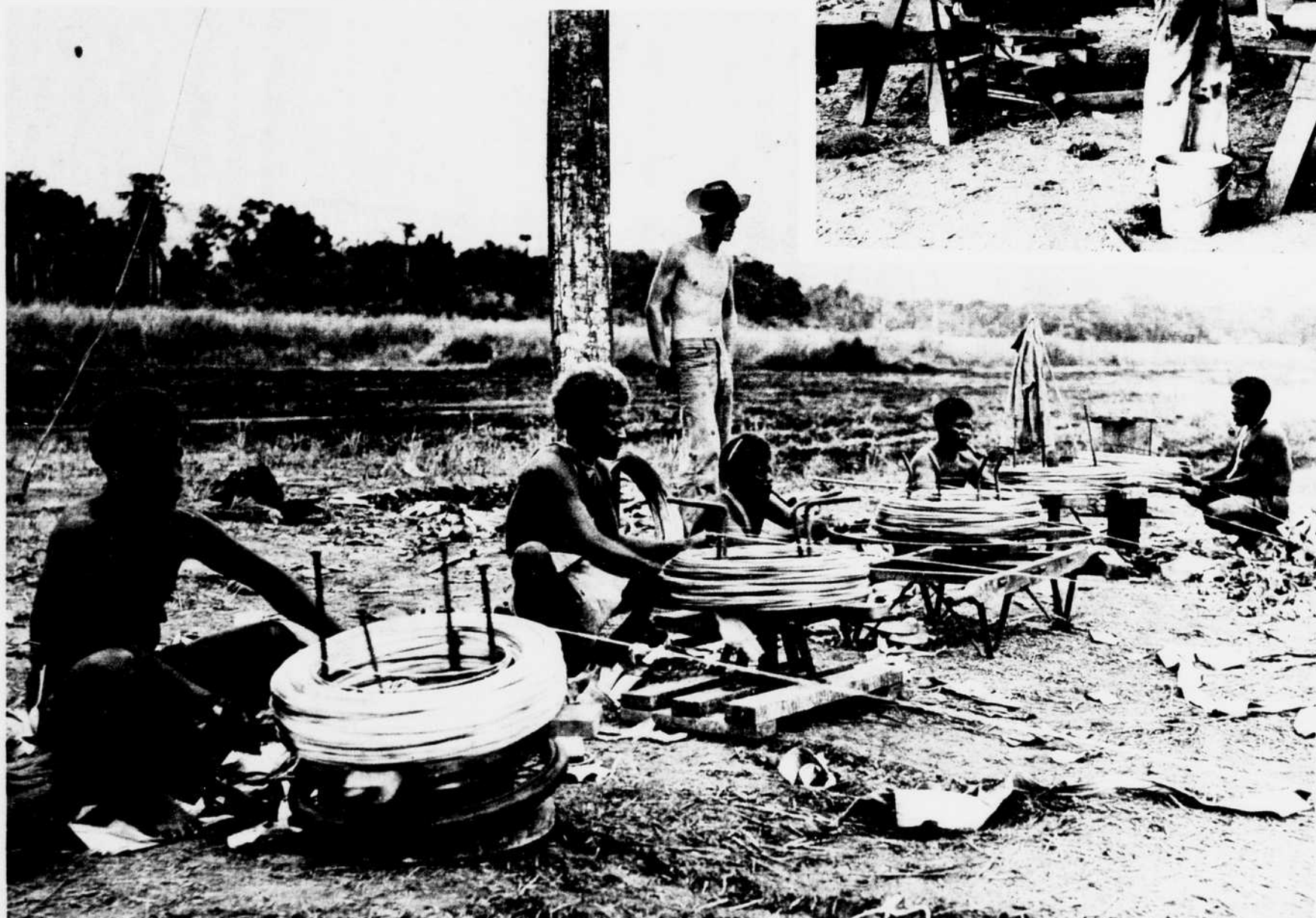
Guadalcanal natives help Marines build more telephone lines on the island. They are tending the reels which pay out the copper wire as it is drawn over the crossarms of new poles.
