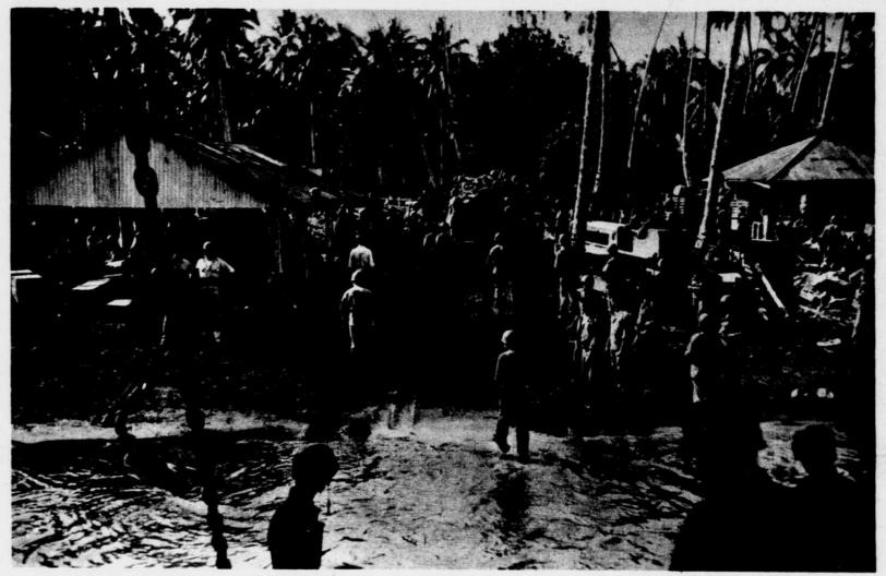
Here marines roll a big gun ashore on Rendova Island. Steel mats were laid across the water gap from the landing craft and on up the soft beach to support the weight of the gun that was soon to join in the shelling of Munda Paint.
