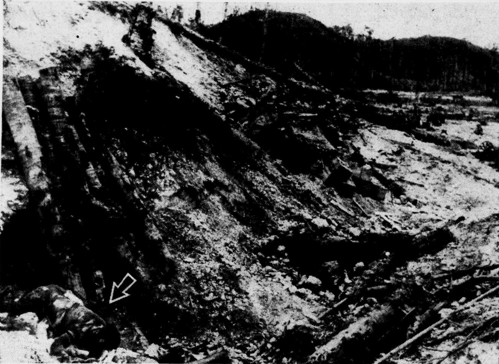
MUNDA.—STRONGPOINT THAT DIDN'T HOLD—Here are two tunnel entrances to Kokengolo Hill, in the center of Munda airfield, where the Japanese put up a last-ditch stand. They dug into the coral hill and were wiped out by Yankee bombs and shells. Bibilo Hill, scene of a bloody battle before Munda finally fell, is in the background. A dead Jap soldier (arrow) lies before the entrance to one of the tunnels.
