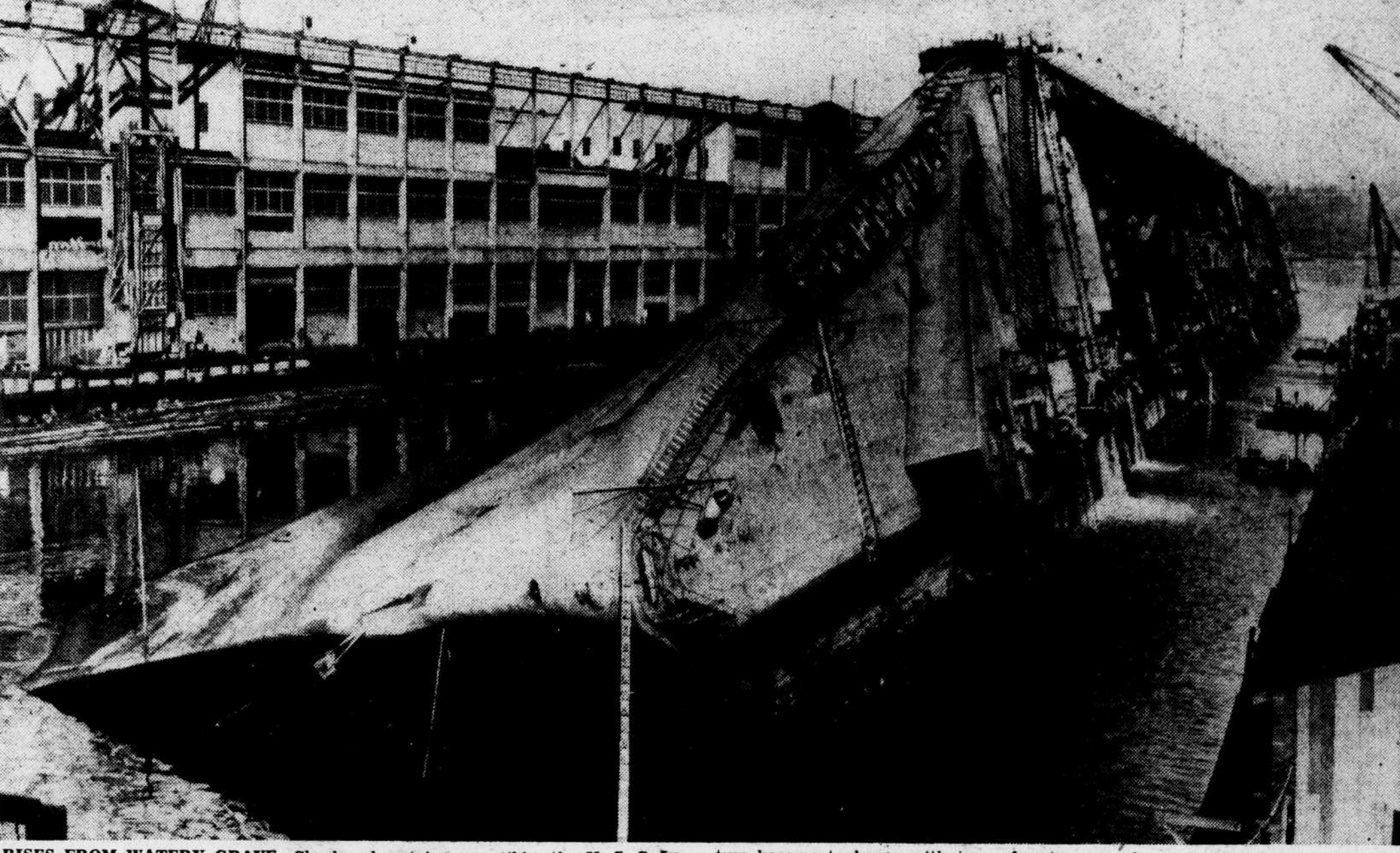
RISES FROM WATERY GRAVE—Slowly, almost imperceptibly, the U. S. S. Lafayette, the former French liner Normandie, today began to right itself at the Hudson River pier. She rolled on her side February 9, 1942, after her superstructure became topheavy with tons of water poured on a raging fire. Note water pouring from her hull.
