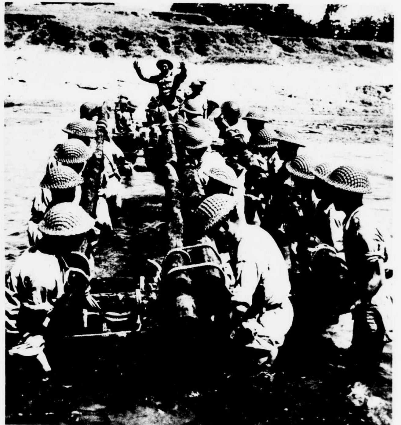
Engineers of the Chinese Expeditionary Forces—which as such probably are destined to help drive the Japs out of Burma and then out of China—build a bridge as part of their training in India. Capt. Sun (hands upraised in background) directs the placement of the center span.
