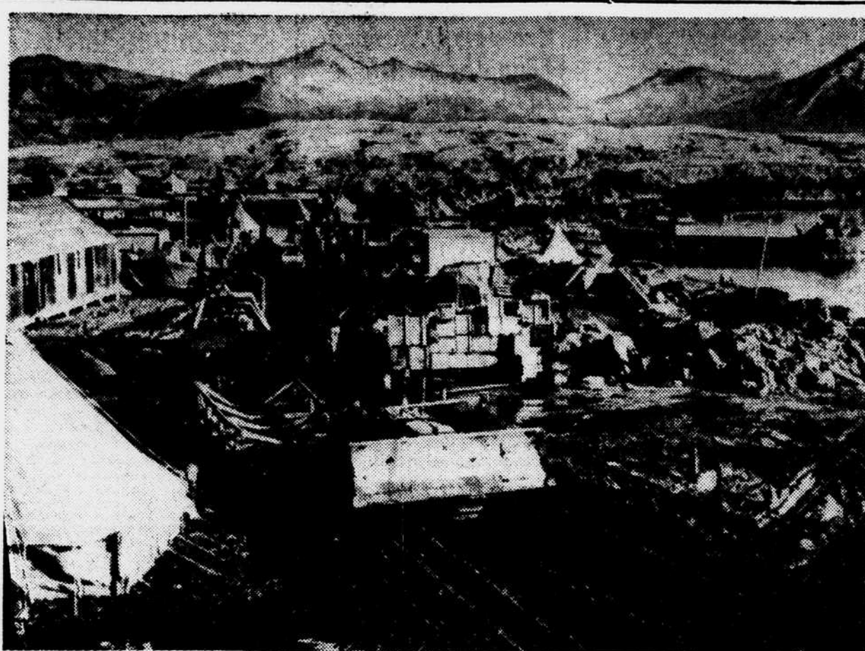
"MAIN STREET," ATTU—Labor battalions have taken over on Attu Island, westernmost of the Aleutians, which was wrested from the Japs, and are busy with hammer, saw and bulldozer. Here a bulldozer smooths the mud-rutted "main street" between rows of tents and the supply-laden waterfront with landing barges along the shore.
