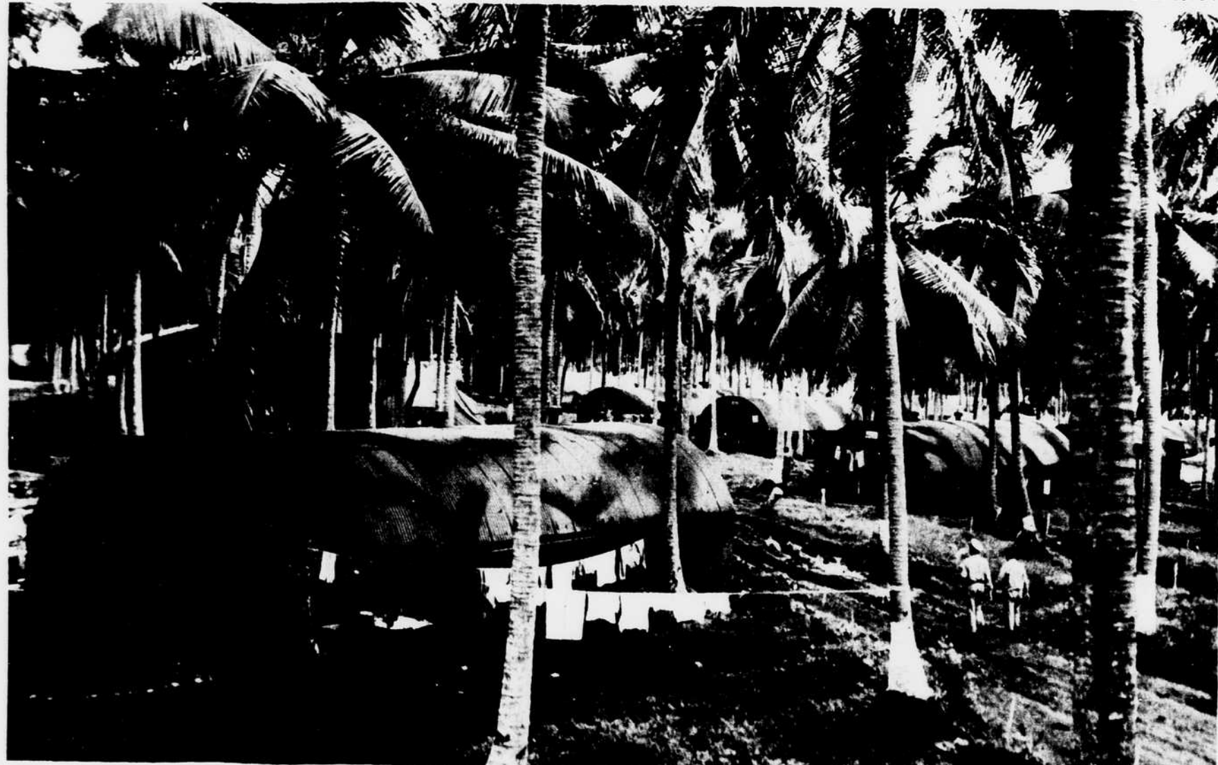
Corrugated metal buildings of the base hospital are wide-spaced under a cool canopy of coconut palms. This "prefabricated" type of building helped the construction battalions do an almost overnight job in establishing the entire center.
