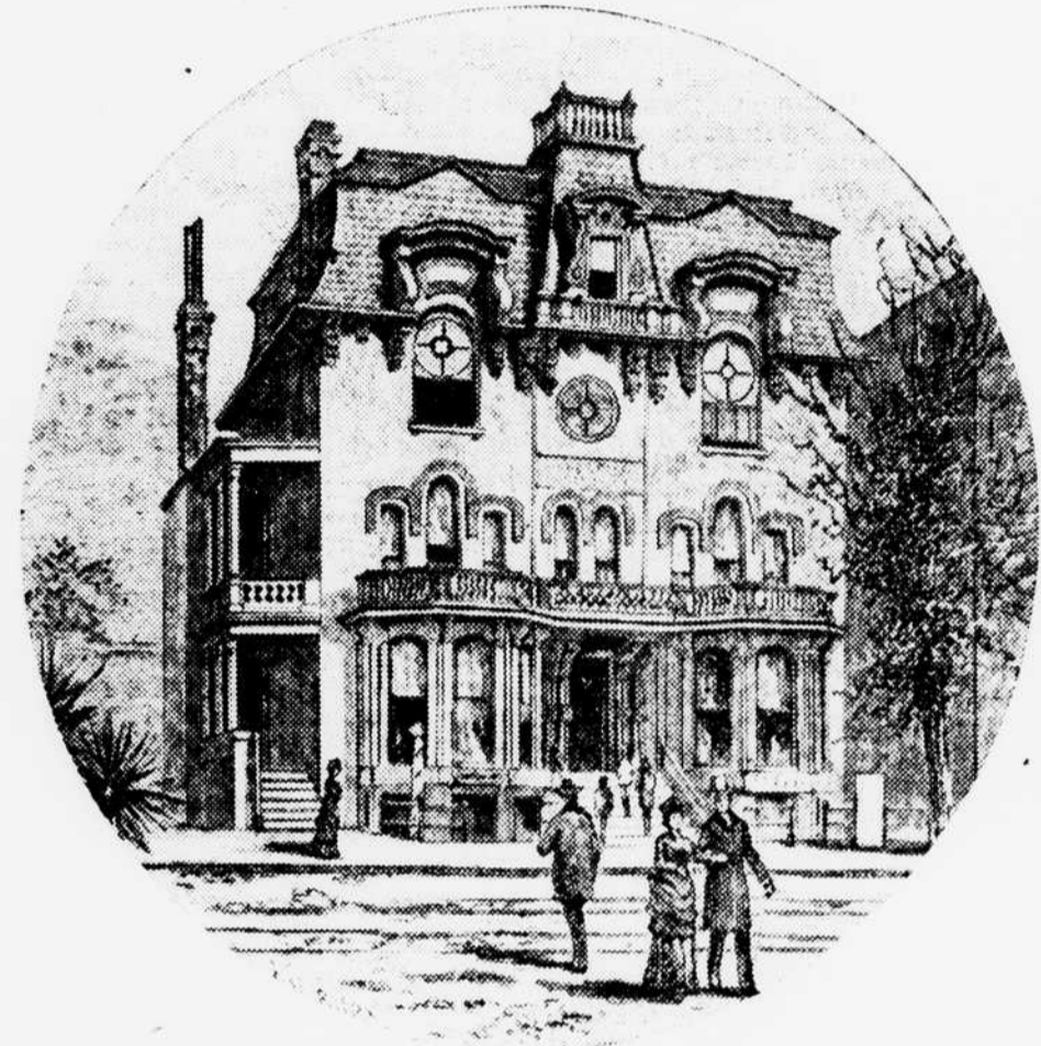
Chamberlin Clubhouse, once the home of the YMCA.
