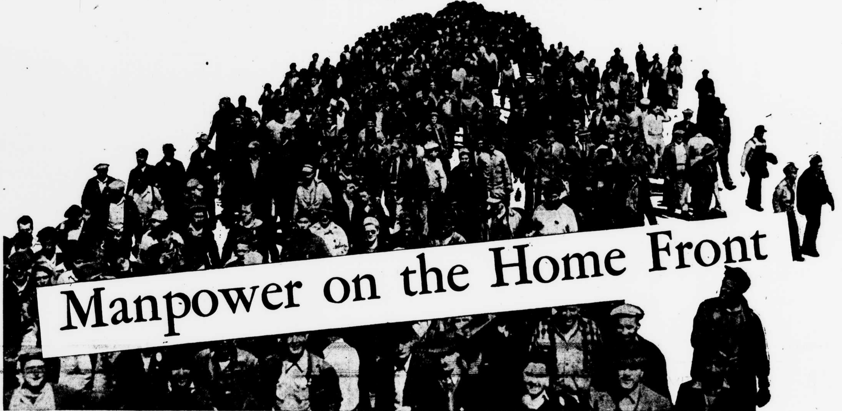
Thousands of men arriving for work in a Bethlehem shipyard. Down this yard's busy shipways slide many of the nation's cruisers, destroyers and aircraft carriers. Bethlehem repeatedly has made records for delivering vessels well ahead of schedule.
