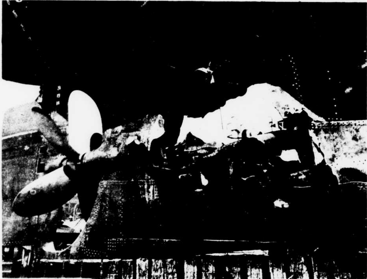
A ship isn't out till it's down! That's the guiding spirit by which this ship was returned to service after a torpedo had torn entirely through its lower stern. It was repaired by the Todd Shipyards Corporation, which then released the picture of the damage.
