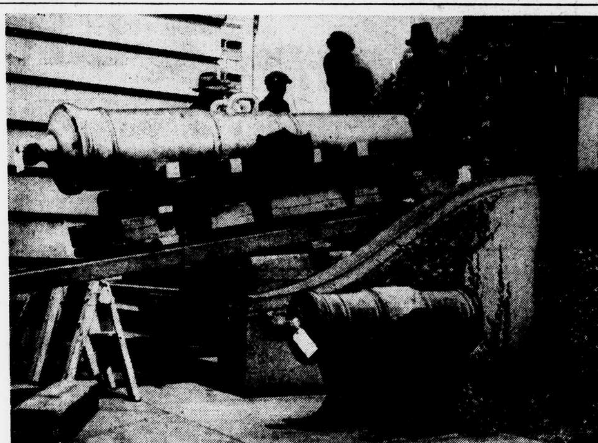
HISTORIC CANNON LEAVE OLD SETTING—Workmen are shown removing one of the 29 historic cannon around the State Department Building as it starts on its way to the Navy Yard to be melted down into bronze. Nineteen will be preserved in other settings. The picture was taken from the north side of the building. (Story on Page A-1)
