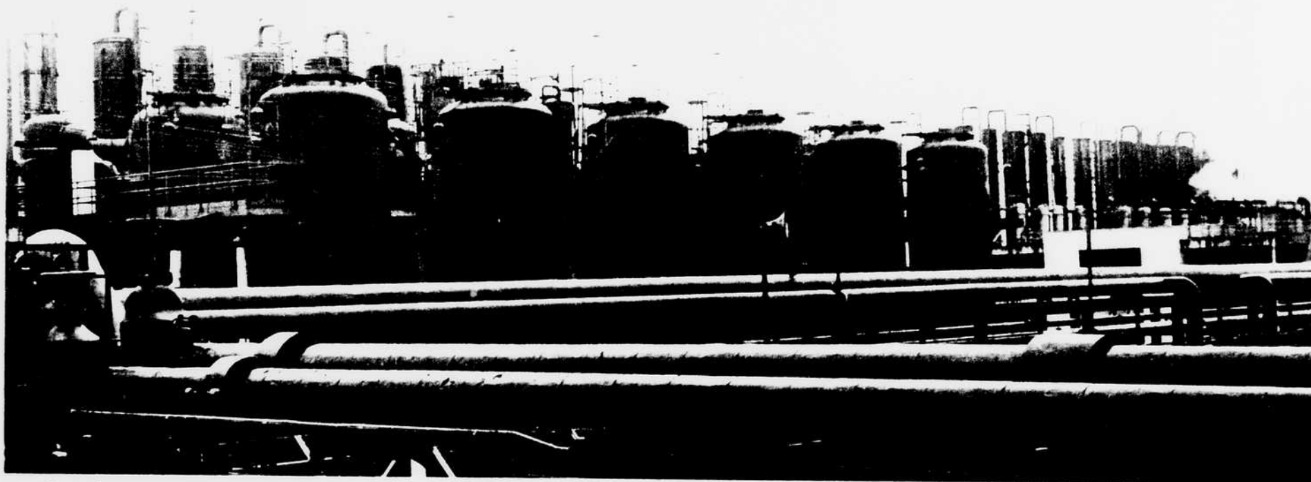
Pipes feed the rubber-making chemicals to the adjoining plant of the United States Rubber Co. In 36 hours of combining and processing in the polymerization plant the butadiene and styrene become synthetic rubber.
