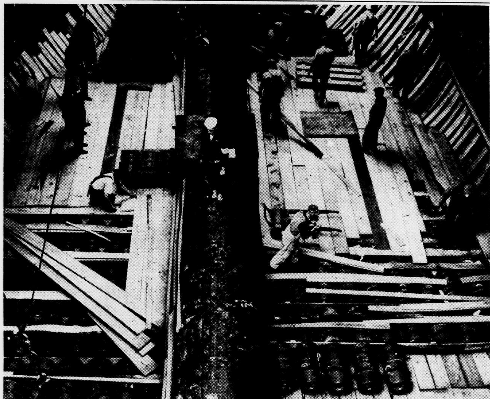
WALKING ON DEATH —Deep in the hold of an Allied ammunition ship, workmen finish the flooring over a layer of 2,000-pound bombs. Every action in the loading of ammunition in the highly vulnerable ship is watched by Coast Guardsmen, who guard against sabotage and enforce safety regulations. —Coast Guard Photo.
