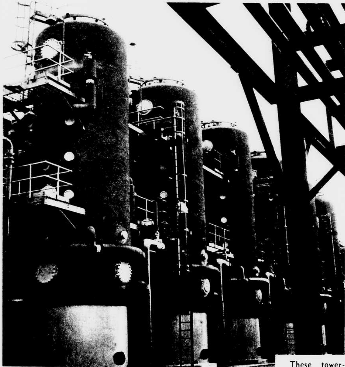
These towering steel chambers are the converters in which grain alcohol is converted into butadiene.
