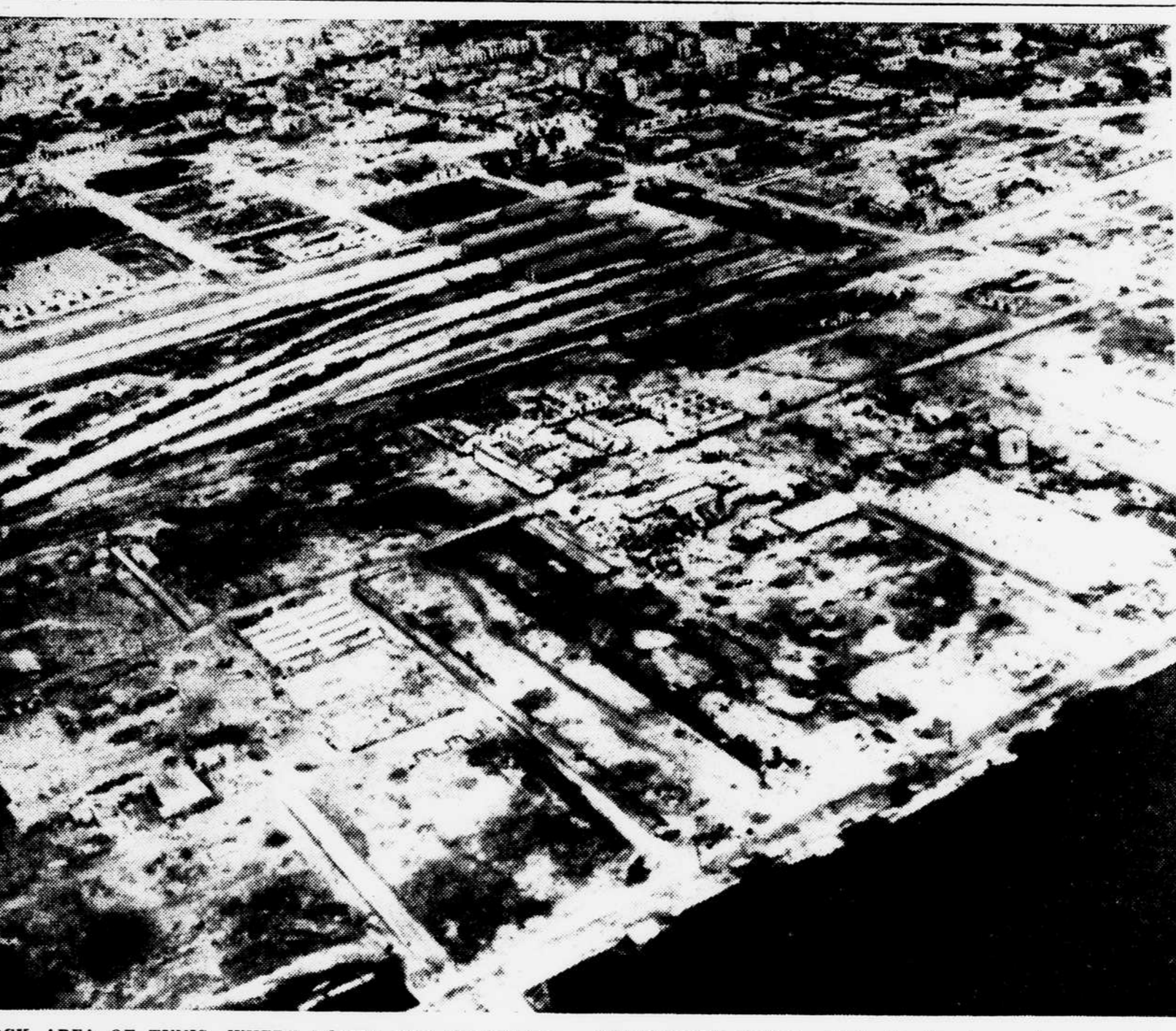
DOCK AREA OF TUNIS—WHERE BOMBS HIT—Devastation by Allied bombs in dock area of Tunis is evident in this air view taken by RAF after the city had been occupied by Allied forces.
