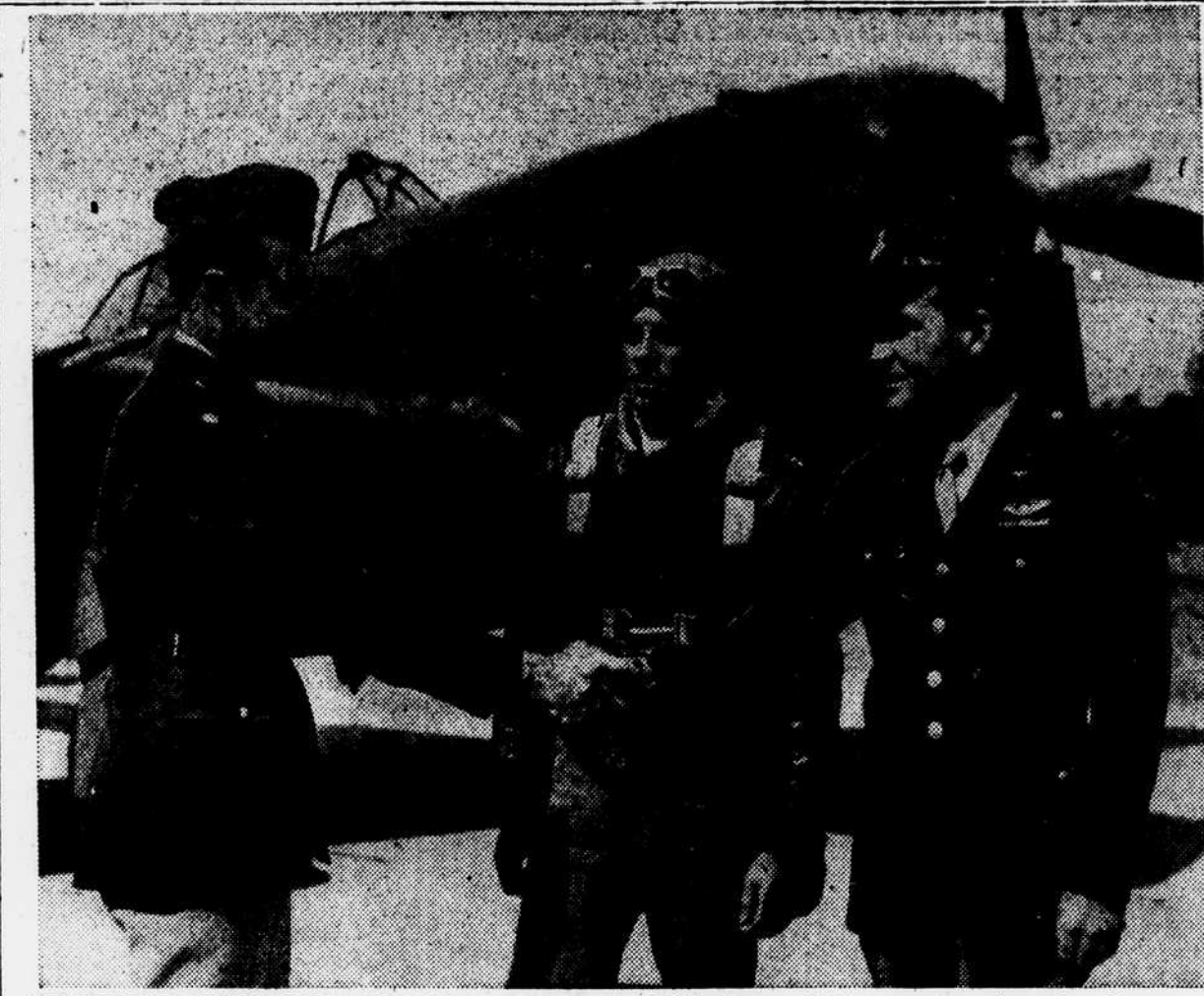
AIR FORCE TAKES OVER AIRPORT—Maj. H. D. Nottingham (left), area engineer in charge of construction at the new Army airfield at Camp Springs, Md., shown yesterday as he turned over military operation of the airfield to Capt. A. W. Salter, Jr., commanding officer of the base. Looking on is Capt. D. A. Younglass, squadron commander, who landed the first pursuit plane. The plane is shown in background.
