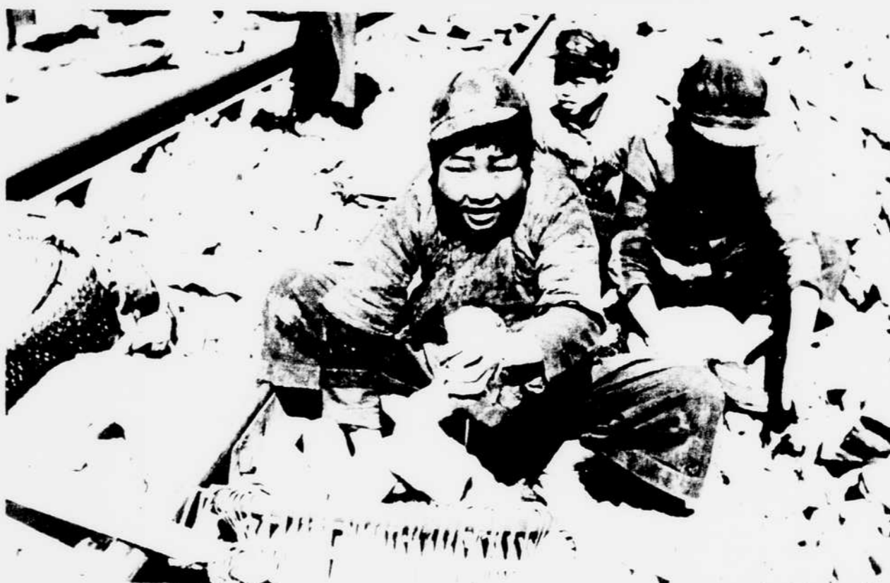
Child labor in China seems to be happy labor—when it's building a new railroad to serve Free China. These youngsters are breaking stone for the roadbed. Children are doing much of this tedious hand labor.
