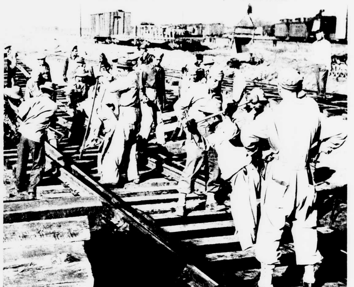
They're in the Army, but they're still railroadin'. Men of the Railway Operating Battalion at Fort Sam Houston, Tex., more than 90 per cent of them former rail workers, train as a smoothly organized force to do everything from laying track, as they are doing here, to operating a complete rail system that may be taken over by the Army anywhere in the world.
