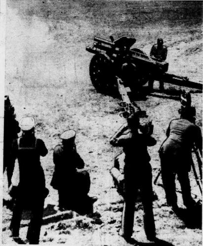
GERMAN GUN TESTED-A German 105-mm. howitzer, captured and brought to the United States for study and comparison with American arms, was fired at the proving center grounds at Aberdeen, Md., under the eyes of photographers and Army officers in an especially-arranged demonstration. It was fired as part of a test of enemy armament arranged by Lt. Col. G. B. Jarrett, chief of the foreign materiel branch of the center.
