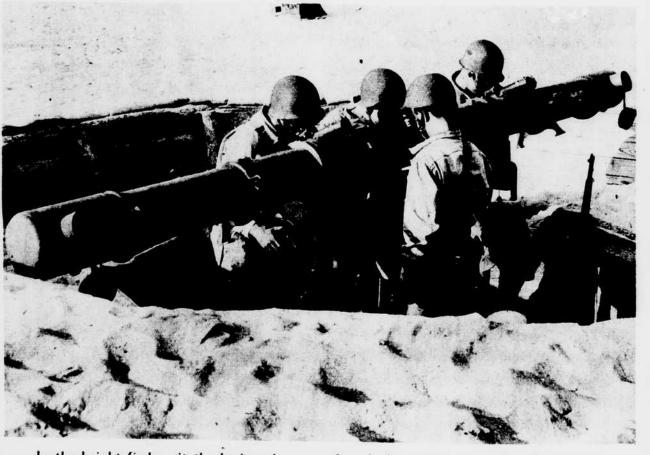
In the height finder pit the horizon is scanned and the target located. This station is tied-in with the electrically-operated mechanism that aims the gun. The man on the right of the instrument is the elevation reader. Others, left to right, are the azimuth setter, the observer, who moves the finder to the target position, and the elevation setter.
