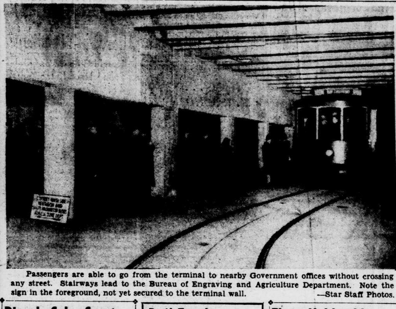
Passengers are able to go from the terminal to nearby Government offices without crossing any street. Stairways lead to the Bureau of Engraving and Agriculture Department. Note the sign in the foreground, not yet secured to the terminal wall.
