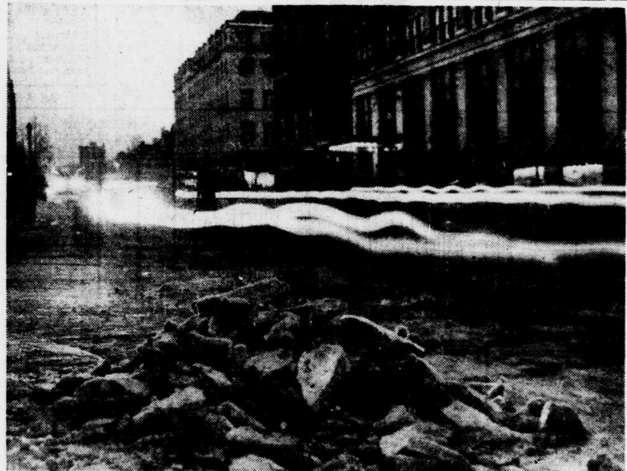
STORM BRINGS BACK CORDUROY ROADS—This time exposure of headlights on an automobile as it bounced across F street in the downtown area gives an idea of the conditions brought about as spinning tires wore holes in the icy surface. Also shown are the lights of a bus as the driver pulled to the right to avoid some of the deeper ruts.
