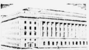
U. S. COMMERCE BLDG. IS 2 BLOCKS FROM RALEIGH
