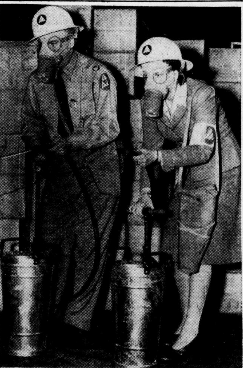
READY FOR ANYTHING—George E. Cox, first assistant deputy warden and training director of the Dupont area, and Kathryn Gailher are shown trying out some of the area's allotment of pump tanks and gas masks which just arrived. Thousands of the pump tanks were shipped here yesterday and more are due today. Unlike the stirrup pumps, these pump tanks have a five-gallon pail attached to the pump. They will be distributed to sector posts for use in combating fires.
