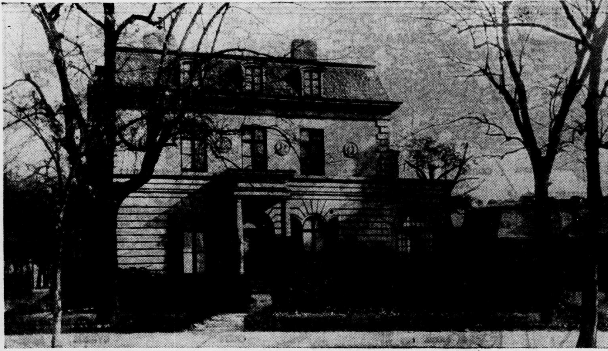
Residence at the southeast corner of Vermont avenue and N street built by Gen. Montgomery C. Meigs and which, in 1905, became the property of Frank B. Noyes, president of The Evening Star Newspaper Co. —Tebbs & Knell Photo.
