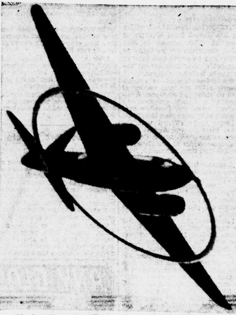
The hooplike device fitted on this Wellington bomber was the "secret weapon" adopted by the British early in the war for exploding magnetic mines from the air. Mine-sweeping from the air is described as hard and hazardous in the new British book, "Coastal Command," in which these pictures are part of a series not previously released.
