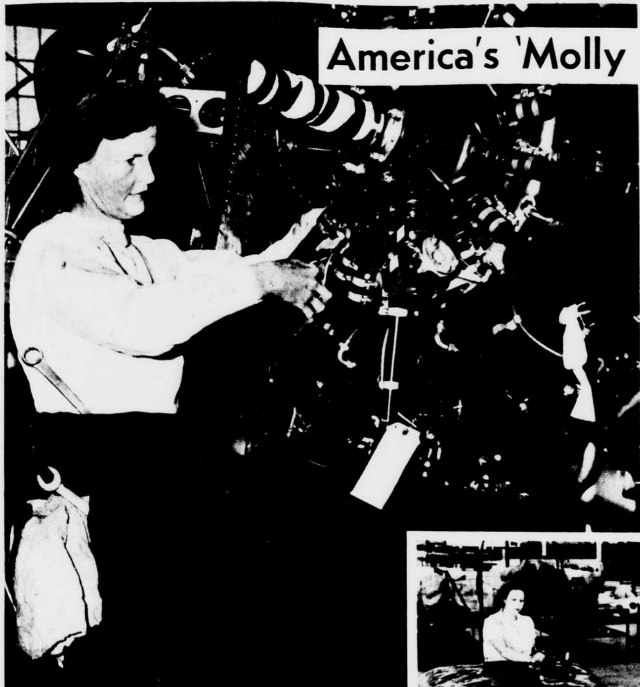
There's no play-acting about the maintenance job Mrs. Jessie Attaway does on advanced training planes at the Blackland Army Flying School, Waco, Texas. Here she's replacing an engine push rod.
