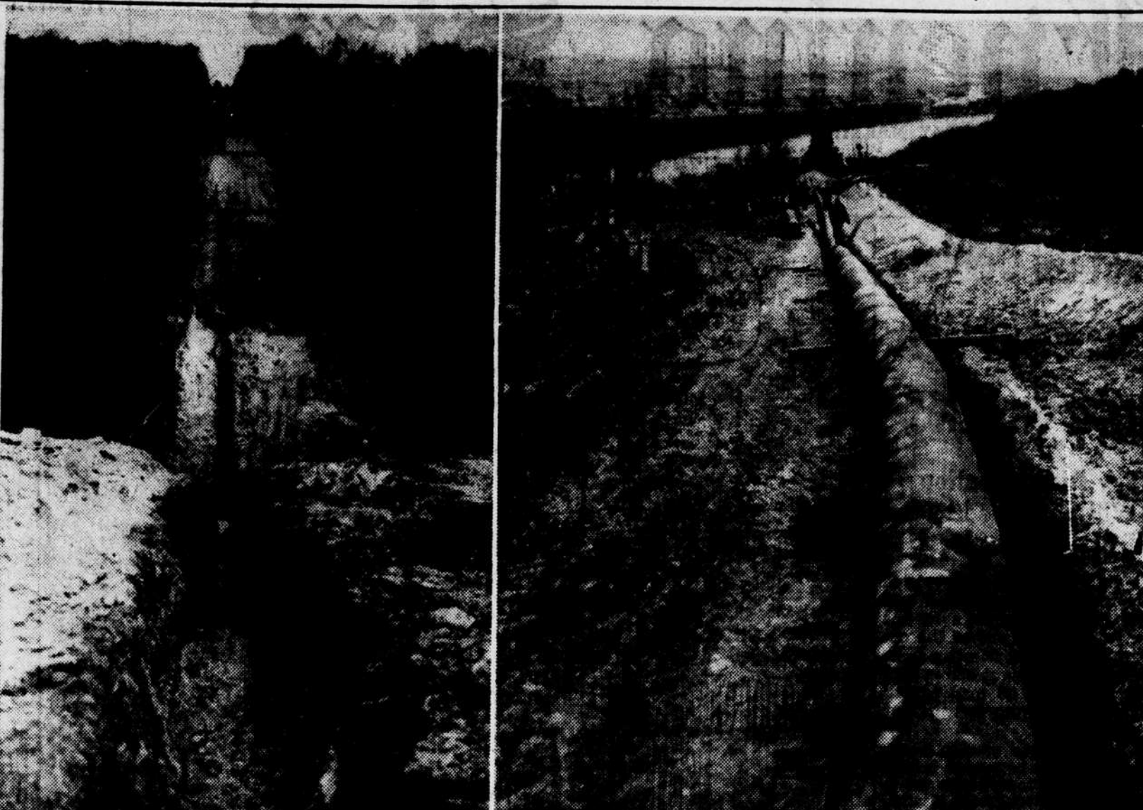
OIL PIPELINE STRETCHES EASTWARD—Work is under way on the Eastern section of the "Big Inch," the world's largest oil-carrying pipeline, on which construction is being pushed to help ease the critical fuel shortage. The photo, taken near York, Pa., shows the ditch for the pipe being dug under difficulties because of woods, rock beds and rolling hills.
