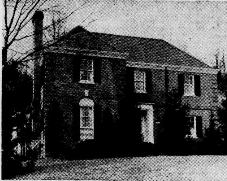
IN ROCK CREEK PARK —This large brick dwelling recently was sold to Lt. Joseph Carey, son of the late Senator Carey of Wyoming, for Col. John Potts. Located at 3514 Williamsburg lane in Rock Creek Park Estates, the transaction was made through the offices of Boss & Phelps.
