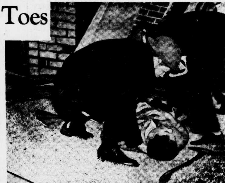
District Civilian Defense workers demonstrate how to remove an injured victim from a collapsed building.
