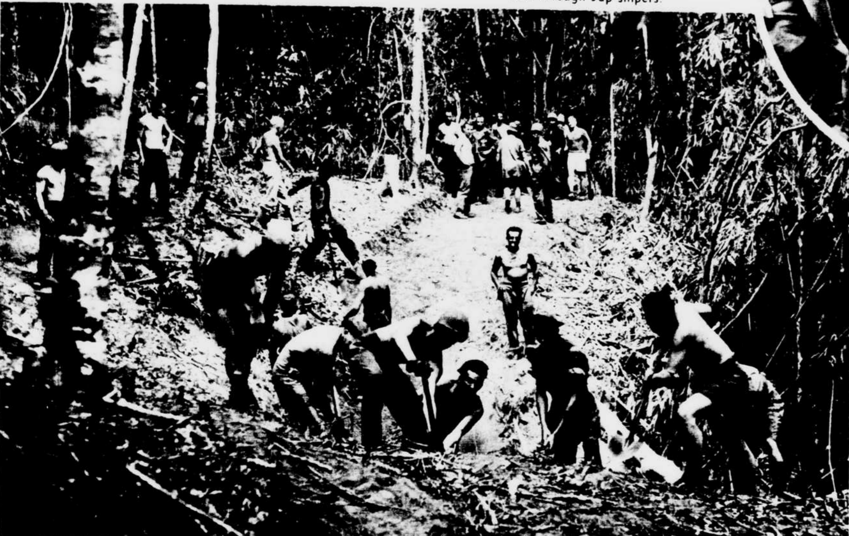
It has been a battle against the jungle as well as the Japs. Through miles of it over the Owen Stanley Mountains troops have hacked and dug a jeep trail to move up supplies for their assault against the Japs in the Buna area. Here's a sample of the toil. A. P. Photos.
