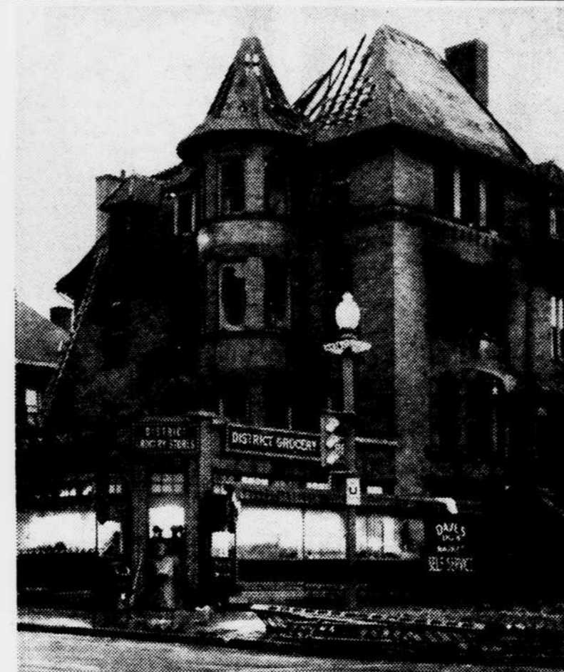
Here is an exterior view of the burned rooming house after fire which killed one person and injured several others.
