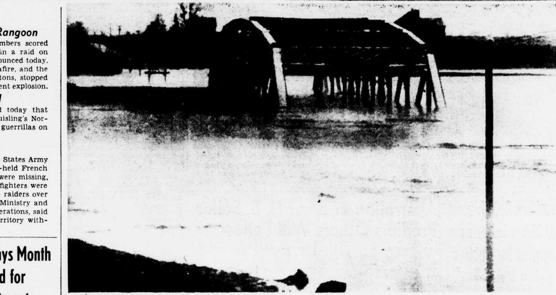
YOUNGSTOWN, OHIO.—FLOODS HARASS OHIO.—Rising waters flooded lowlands in Ohio, Pennsylvania and other States today. Here is what happened to a bridge on the Youngstown-Akron road when the new Berlin Dam, built near Youngstown to store water for Mahoning Valley steel plants, failed to release water as fast as it flowed into a reservoir area.
