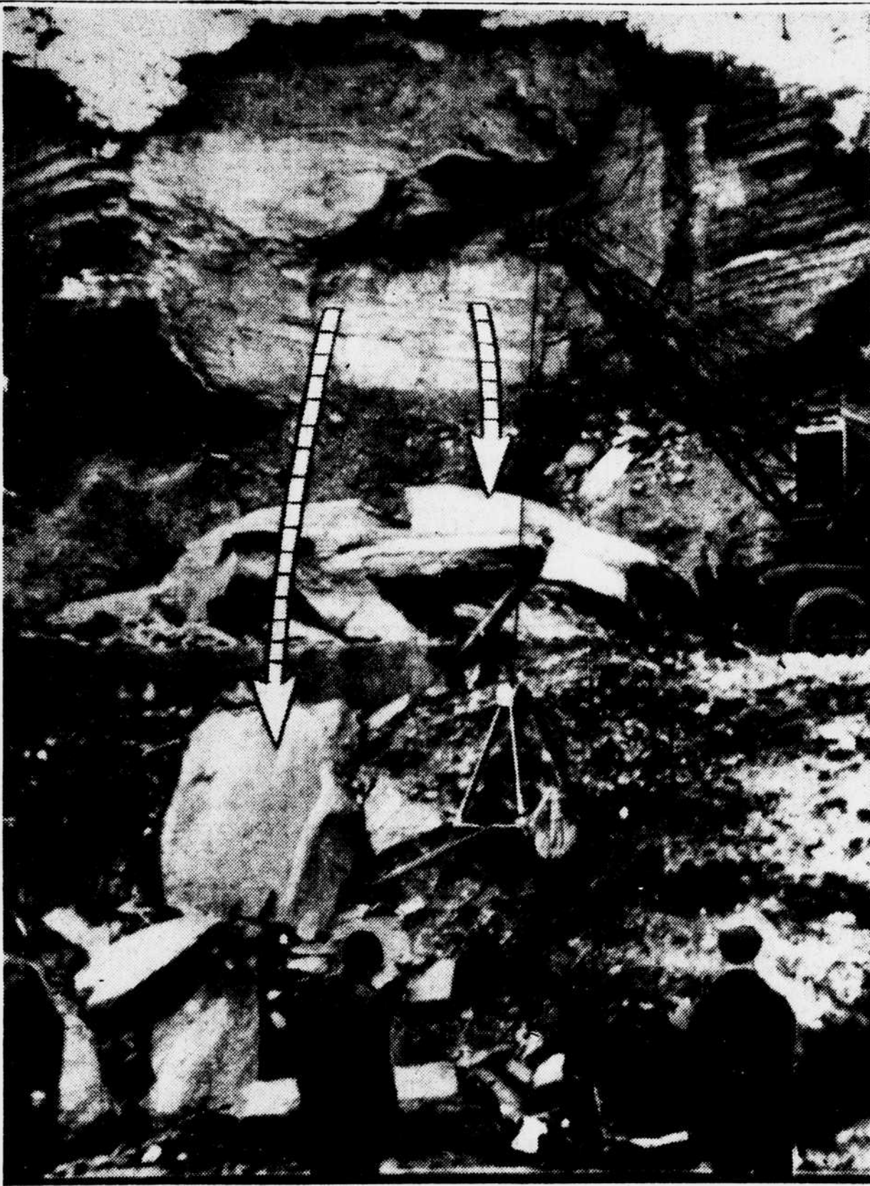
ALIIQUIPPA, PA.—SCENE OF BUS TRAGEDY—A crane is shown removing rock from the road after two huge boulders crashed down on a bus loaded with war workers last night, killing 22 persons. The short arrow shows how the boulders fell from the ledge. The longer arrow is the path of rocks which bounced across the road. (Story on Page A-1.) —A. P. Wirephoto.
