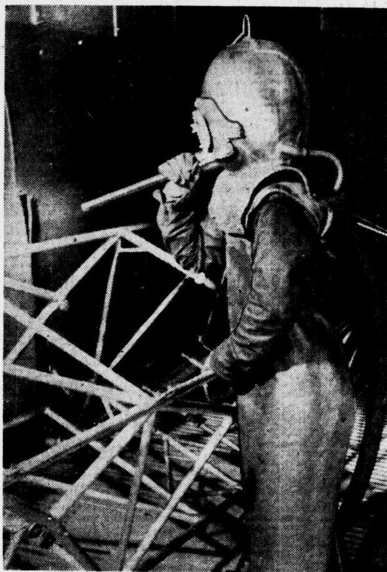
WICHITA, KANS.—DEEP SEA DIVER? GUESS AGAIN —Harry Cline-Smith, sand blaster at the Boeing Airplane Co. plant, swiftly removes scales of dirt from a fuselage with a powerful blasting hose. The headgear weighs 14 pounds and prevents him from inhaling dust particles. —Wide World Photo.
