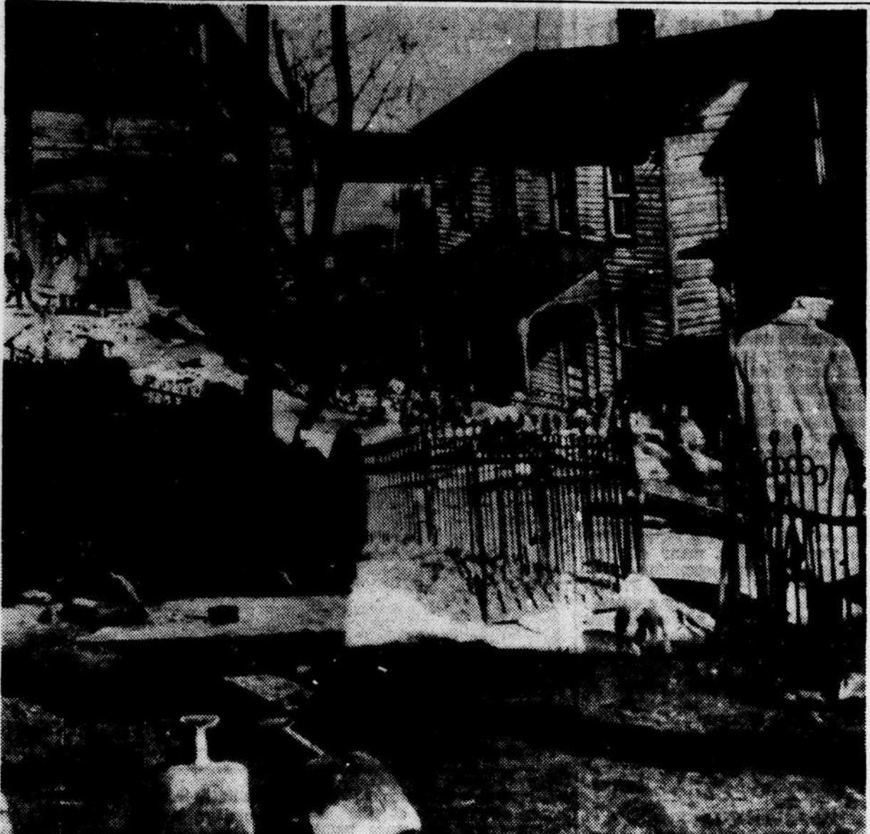
PITSTON, PA.—MINE CAVE-IN DAMAGES HOMES—These houses were among 275 damaged by a mine cave-in under this anthracite town. The center house was at level of foreground before the surface gave way Saturday. In background is demolished concrete structure. Surface cracks in foreground are a foot and a half wide and extend over several blocks. The mine under the town has not been worked for more than 50 years. —A. P. Wirephoto.
