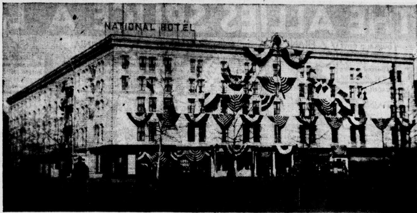
The National Hotel at Sixth street and Pennsylvania avenue, now being demolished, where the District Bar Association was formed in May, 1871.
