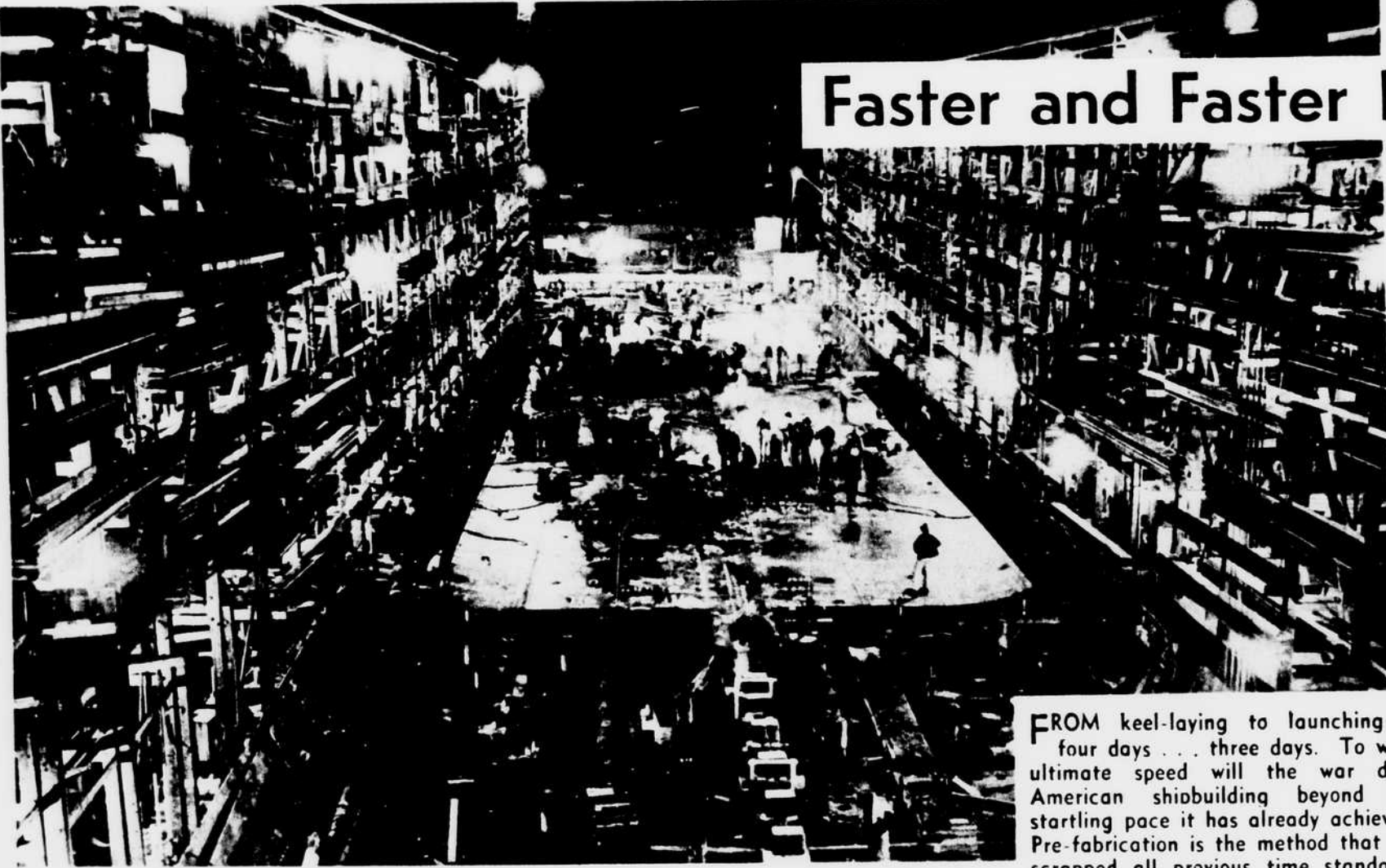
Night lights brighten the scene at the Richmond, Calif., yards as keel plates are welded in the early hour stages of the building of the Liberty ship Robert E. Peary.
