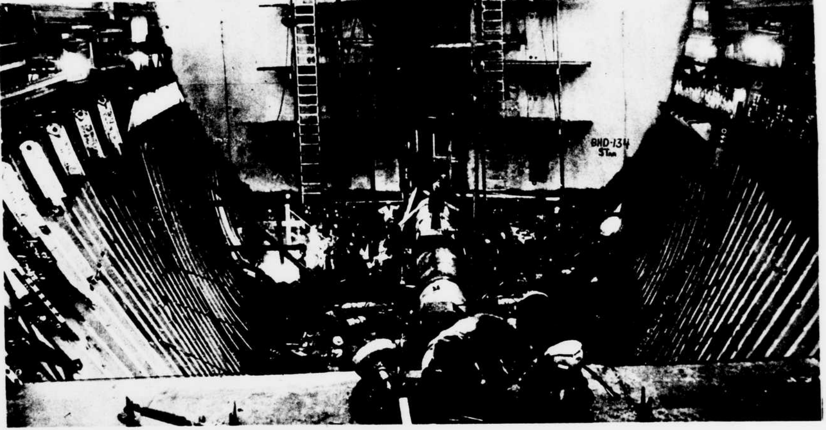
A great bulkhead, complete, is lowered into place in the hull of the Peary which, from the foreground, already is starting to be decked over with less than half the building time elapsed.
