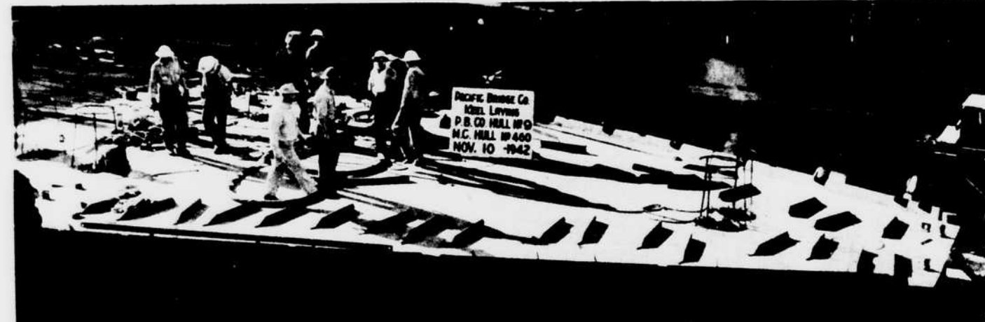
Mr. Kaiser has touched off a hot race in shipbuilding. Eighty hours after this keel of the 8,000-ton freighter Samuel Very was laid at Alameda, Calif., the hull was floated
