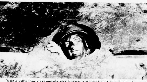
What a wallop those sticky grenades pack is shown in this head-size hole made in tank armor by a practice toss. This is the first of a one-two punch. Next comes the bottled gasoline, tossed in the hole or near it, and survivors in the tank hasten to get out.
