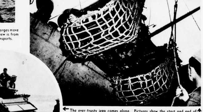
The ever-trusty jeep comes along. Pictures show the start and end of tis trip shoreward. It is slung from ship to barge in cargo nets and drives off the barge into the sea for the beach.
