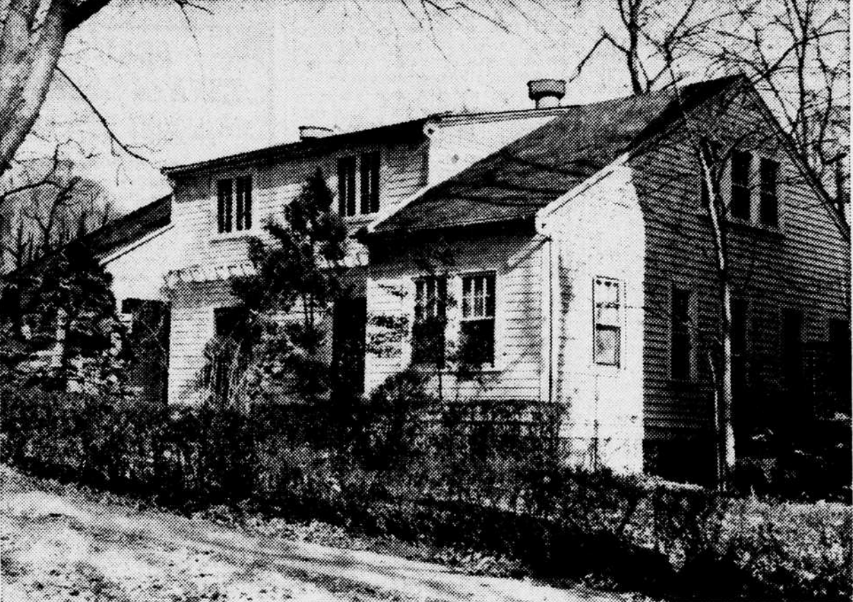
ATTRACTIVE COTTAGE—This home at 2911 Thirty-third place N.W., has been purchased by Mrs. E. Brooke Lee of Silver Spring, Md., from Sidney Paige of New York through the office of Boss & Phelps. The second story is being enlarged and renovated. Mrs. Lee said she bought the cottage as "an investment." —Star Staff Photo.
