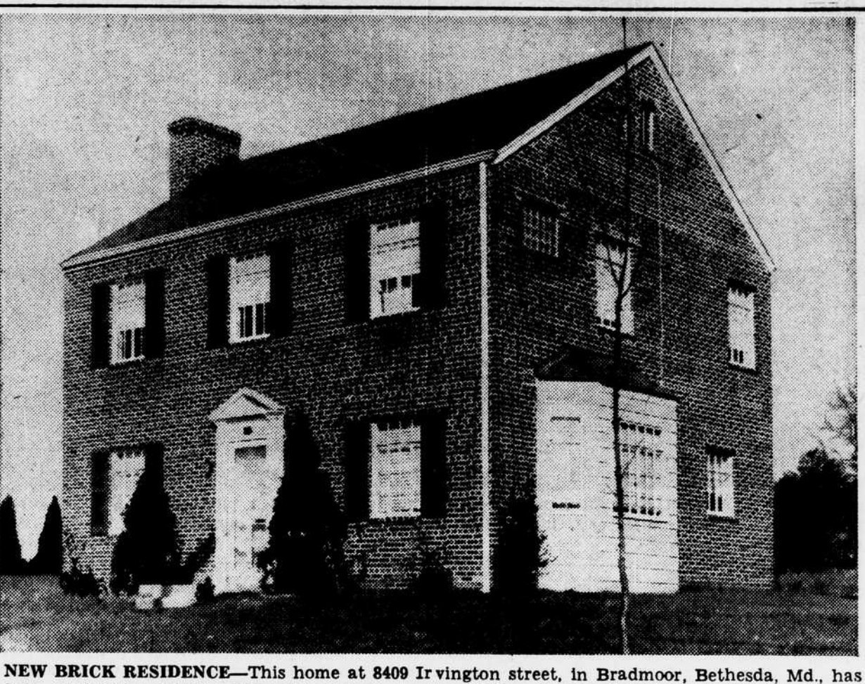
NEW BRICK RESIDENCE—This home at 8409 Irvington street, in Bradmoor, Bethesda, Md., has been sold to Mr. and Mrs. Samuel H. Scheide by the William H. Saunders Co., Inc. It was built by William E. Yost. —Star Staff Photo.
