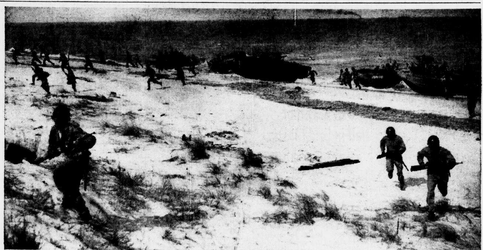
NORFOLK, VA.—NEGRO SEABEES IN ACTION—Their boats pulled up on the beach, Seabees of the Navy's first Negro unit of the construction outfit charge over the sands. They are being taught to work and fight in training courses and maneuvers.
