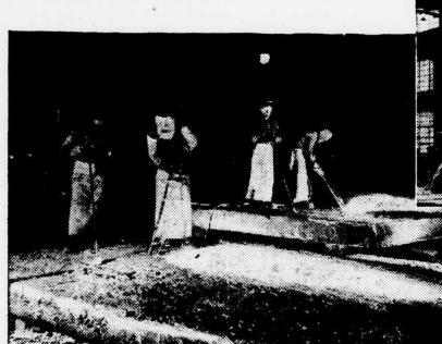
relining and enlarging a blast furnace in record time. Another record relining
