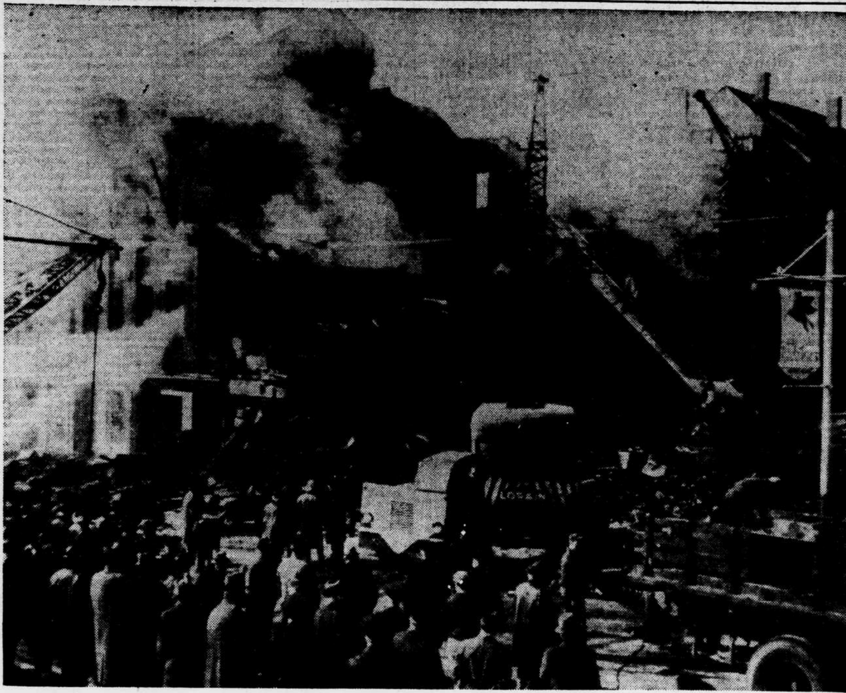
BOSTON.—SIX FIREMEN KILLED IN BUILDING COLLAPSE.— Firemen, police, sailors and shipyard riggers comb the wreckage after the collapse of a brick building wall, which killed six and
