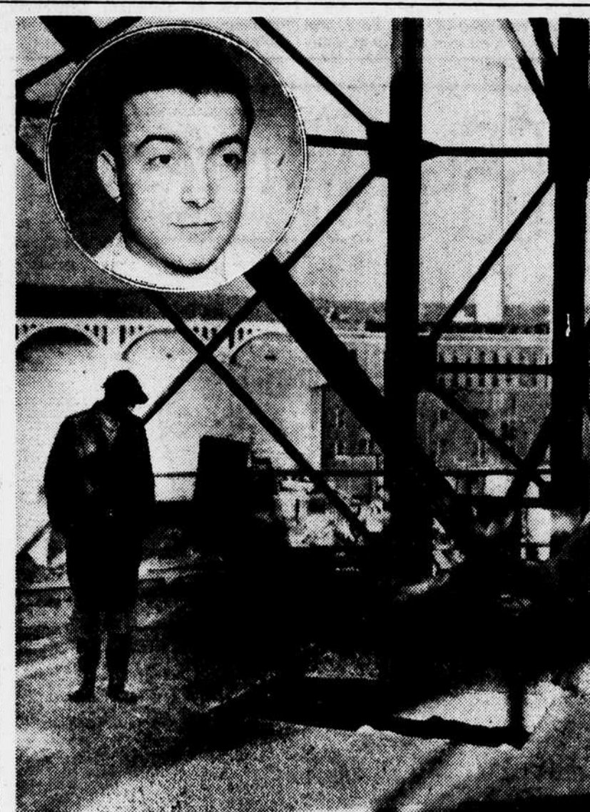
SCENE OF FATAL FALL—The picture at the left shows the opening at the top of the gravel bin at Thirtieth and K streets N.W., into which John E. Fulk, a belt man for the Smoot Sand & Gravel Co., fell to his death early today. In the picture on the right Mr. Fulk's drop of 60 feet inside the bin is traced by a dotted line on the bin's exterior.
