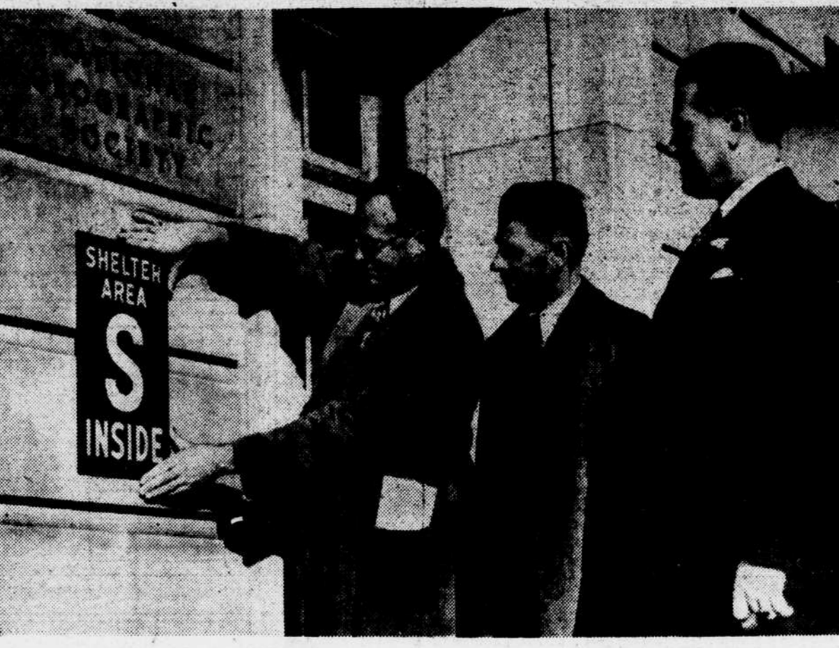
FIRST SHELTER SIGN UP—Passers-by caught on the street during raids or drills will know from this sign that there is shelter within. First sign posted today at the National Geographic Society Building. Shown at the posting are (left to right) A. L. Kundzin, head of the Engineer Department's air-raid shelter survey section; H. C. Kleinstuber, also attached to that section, and Leonard C. Roy, chief shelter warden of the National Geographic Society. —Star Staff Photo.
