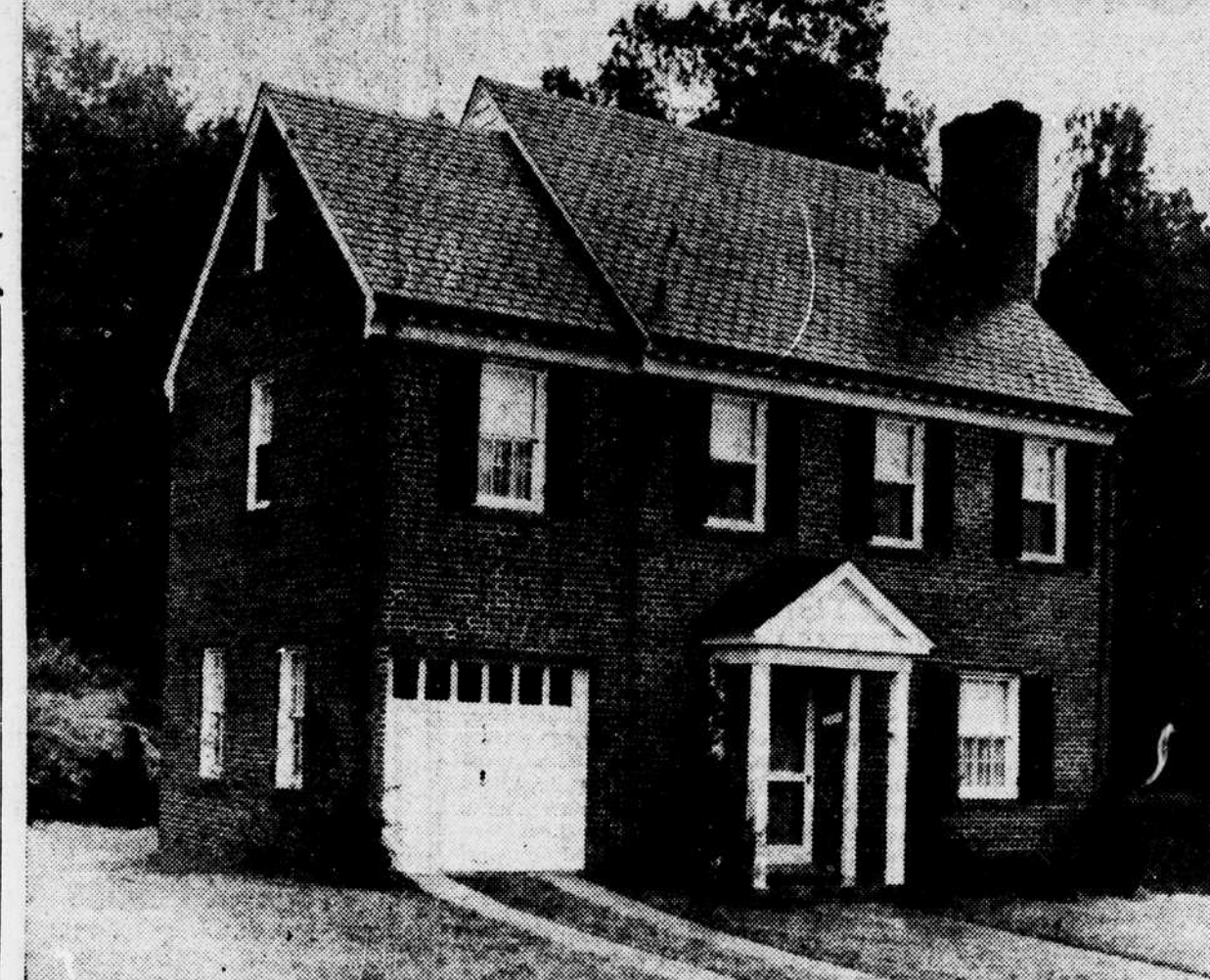
NEW HOME—This delightful brick home has been purchased by Mrs. W. W. Benson through the offices of Leslie D. Messell, real estate broker. Built by B. G. Eastham, it is located at 2914 Legation street N.W.
