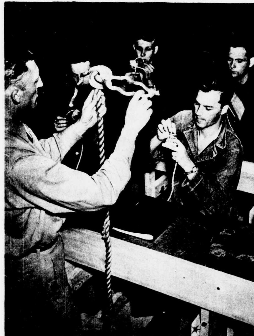
Learning tricky knots is one of their specialties. Here Pvt. Robert Kehr teaches a cordage class of balloon trainees how to make a "monkey's fist," a knot used in rigging a balloon.
