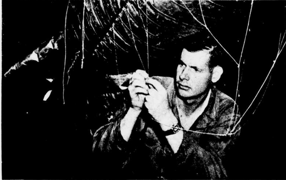
By practice with miniature models, trainees get wise to all the complicated rigging by which a balloon is held captive with equal stress everywhere.
