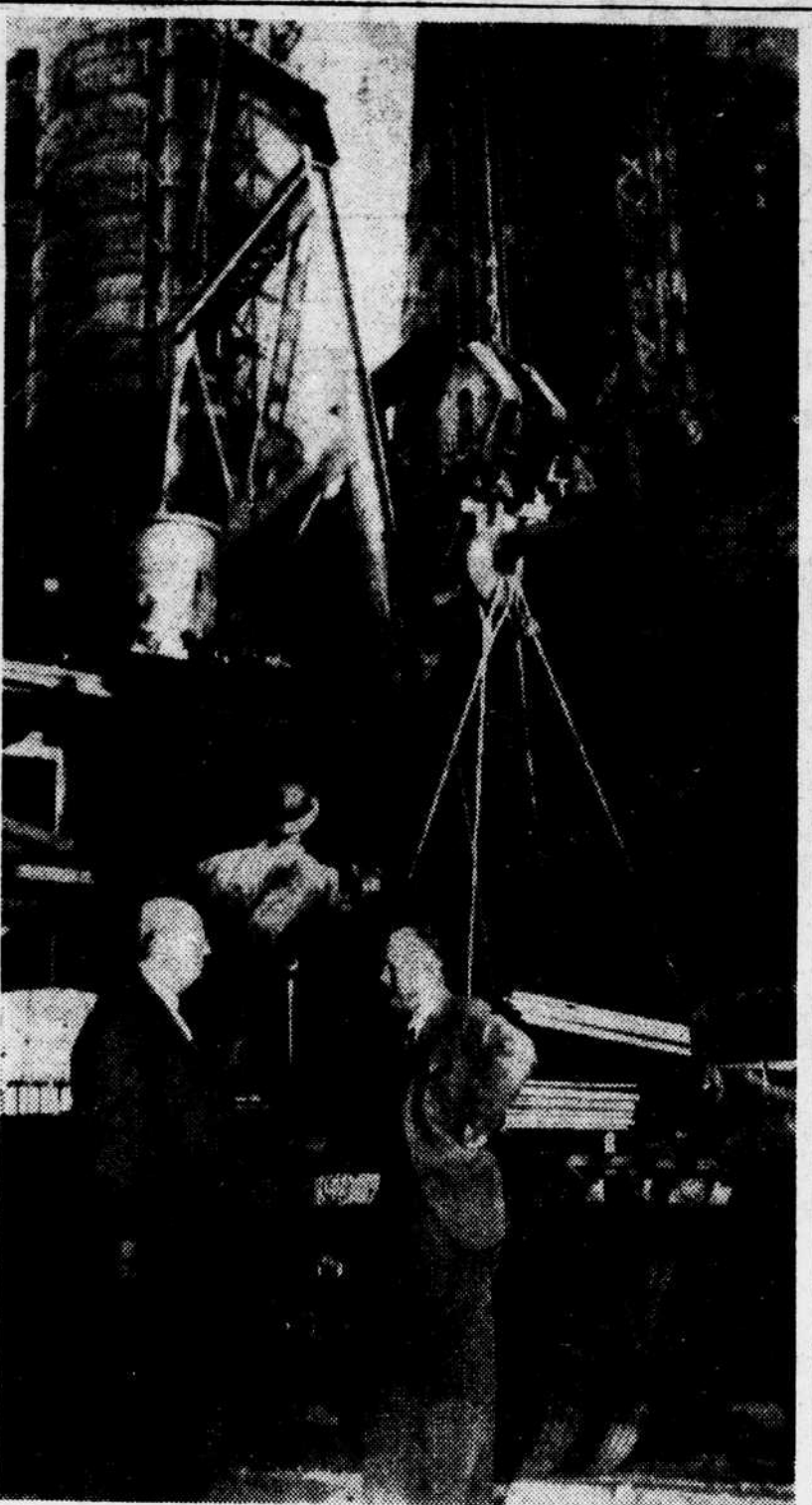
FONTANA, CALIF.—KAISER GETS PROGRESS REPORT—Henry J. Kaiser (left) hears Tom Price, construction manager, describe progress on the new steel mill the industrialist is building near here.
