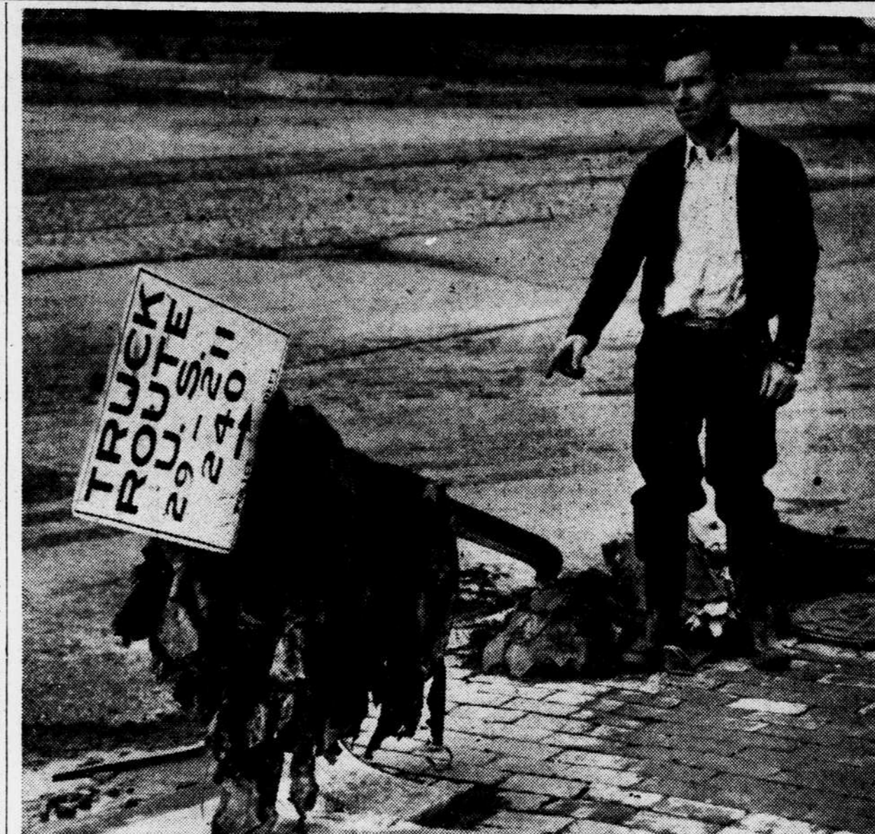
IN FLOOD'S WAKE—So strong was the force of the Potomac River when it swept past the Georgetown water front this traffic direction sign was bent downward. John McRae of Alexandria, Va., points to debris on the marker at Wisconsin avenue and K street N.W.
