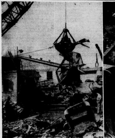
HOW SCRAJ IS PROCESSED-An auto body being hoisted by a crane and dropped into a compressor chamber at the processing plant of Joseph Smith & Sons, 3619 Benning road N.E. The wood and other non-metal parts previously had been removed. This step starts the conversion of bulky junk into material that can be shipped to steel mills.
