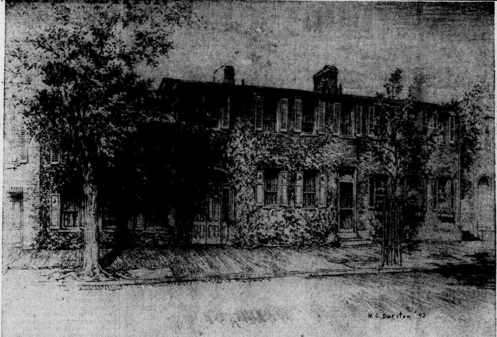
THE "YELLOW" OR "WHITE HORSE" TAVERN—Where a Government official now lives and entertains the leaders of today's democracy, weary travelers used to stop before the United States was born. Built in 1771, it was a prosperous tavern in the days of Georgetown's commercial importance before the seat of the Government was established a little way down the "Potomak" and dwarfed the enterprising little town. Helen Gatch Durston
