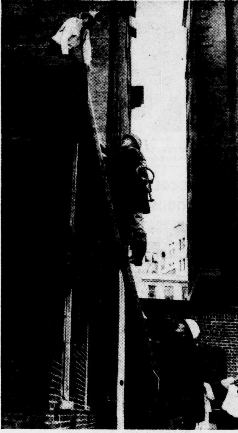
Auxiliary firemen are not coddled by officers of the regular department. Here Theodore J. Heller, on the ladder, and W. M. McIntosh, below, are carrying a line up to Lt. A. E. Bigos of Engine Company No. 1 on the roof.
