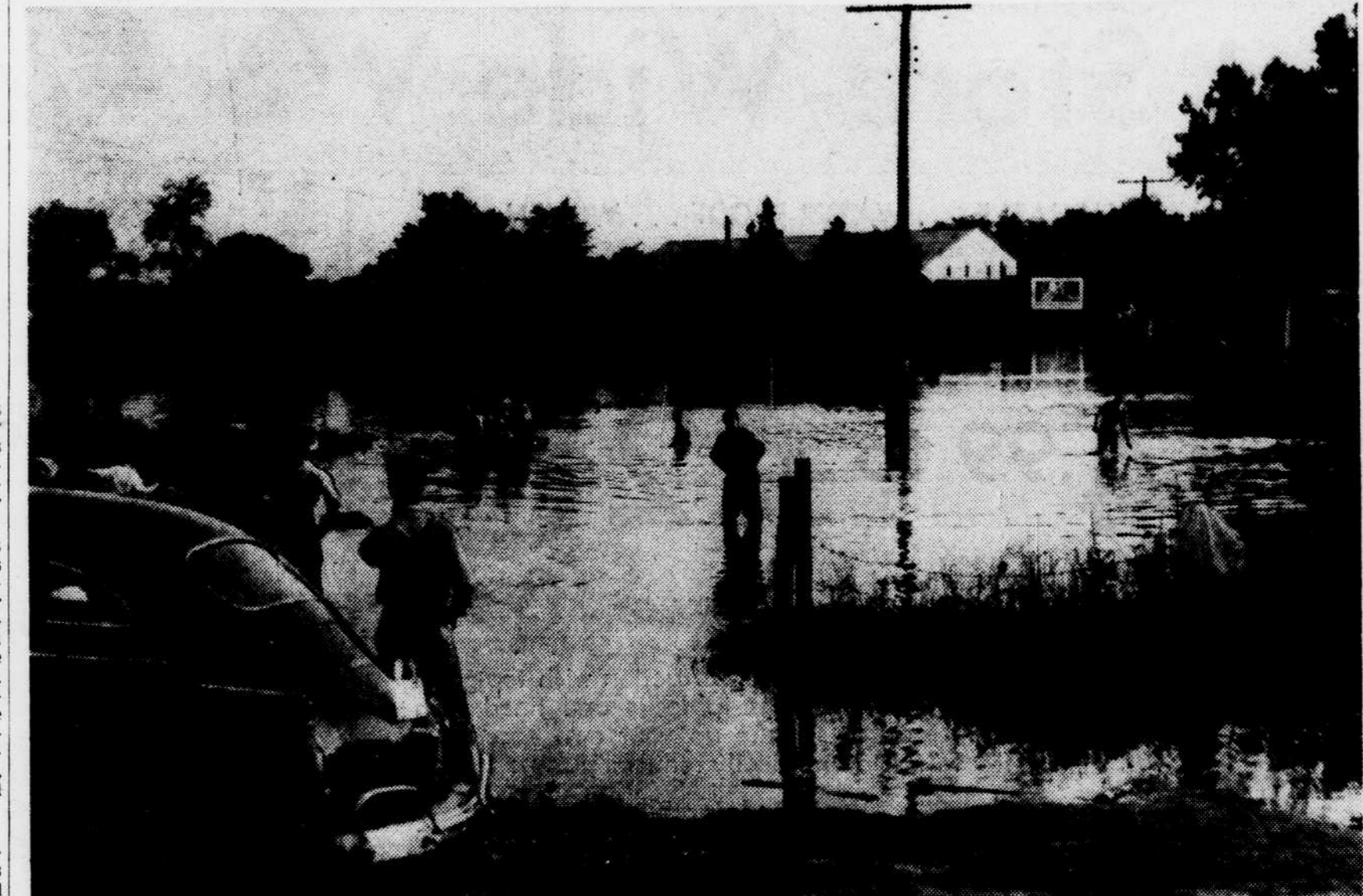
THIS USED TO BE A HIGHWAY—A view of the flooded section of Route 4, just outside of Upper Marlboro, Md., yesterday. More than 5 feet of water, caused by the overflowing of the Collington Branch, covered approximately 1/2 mile of the road, forcing
