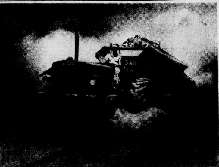
Here's a load of St. Marys County soil being rushed from a runway site to a low spot in a "Eukie" through clouds of dust. The "Eukies" are 150-horsepower Diesel jobs that are able to romp along at 40 miles per hour with a load of 15 cubic yards of soil. By use of caterpillar-drawn elevating graders they can be loaded in slightly more than 1 minute.
